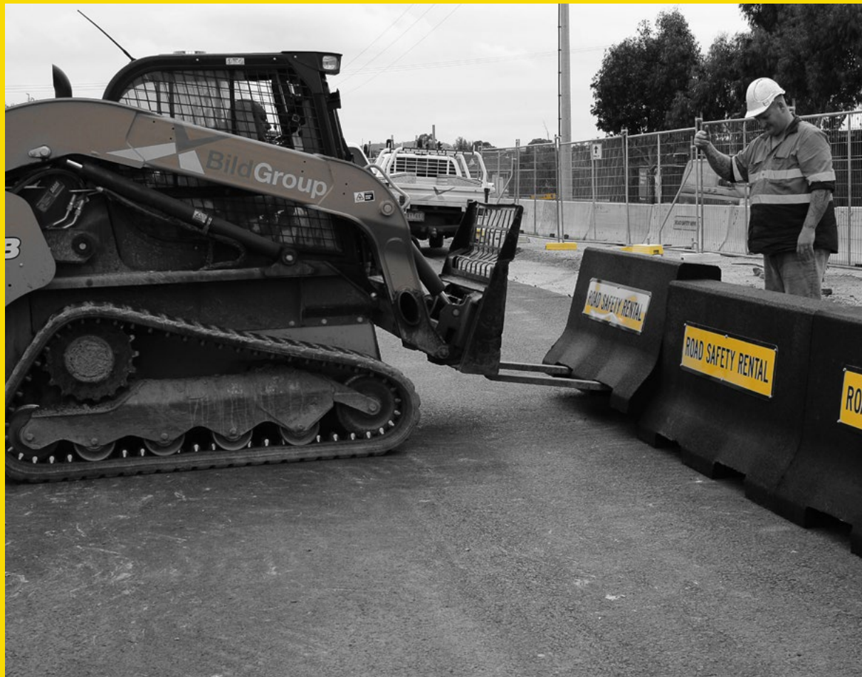
Rubber Guard Barrier being deployed at a Bild Group site, Pakenham, Victoria.
